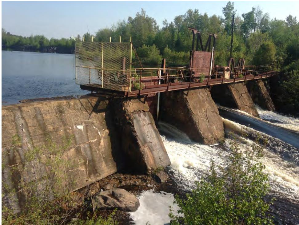
Photo No. 1 – View of downstream face of the dam looking north.
