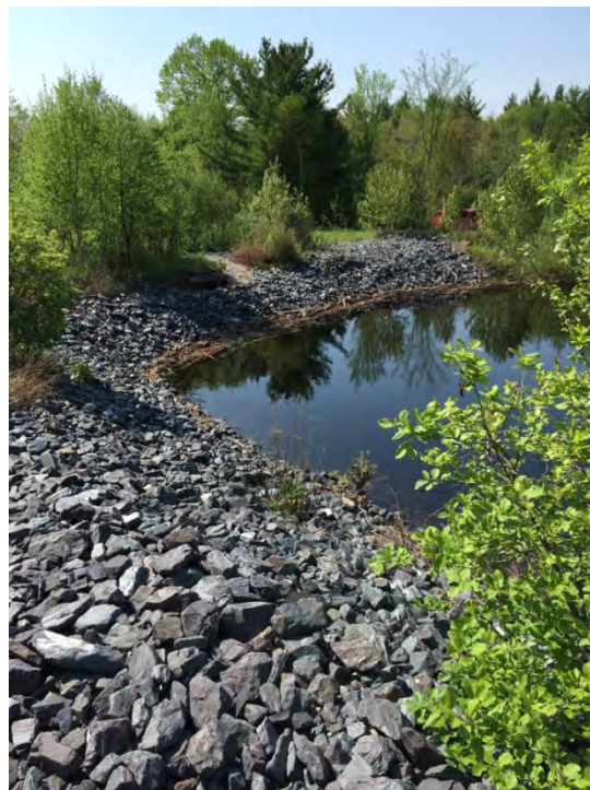
Photo No. 4 – View looking south at the former powerhouse site. Note the riprap armored slopes of the former intake canal.
