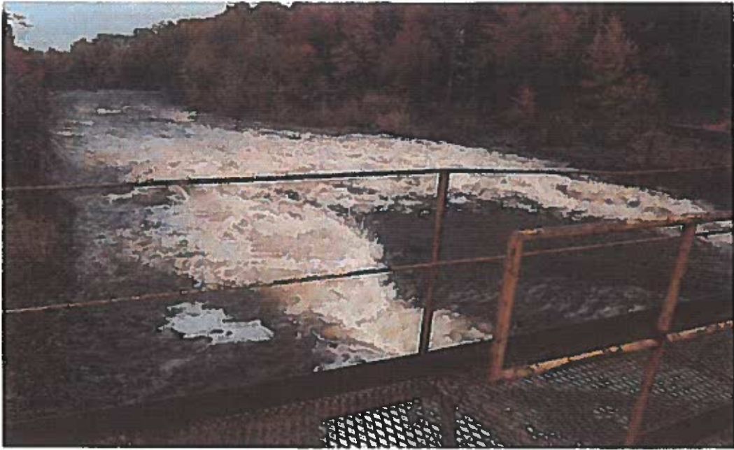
View from dam.
