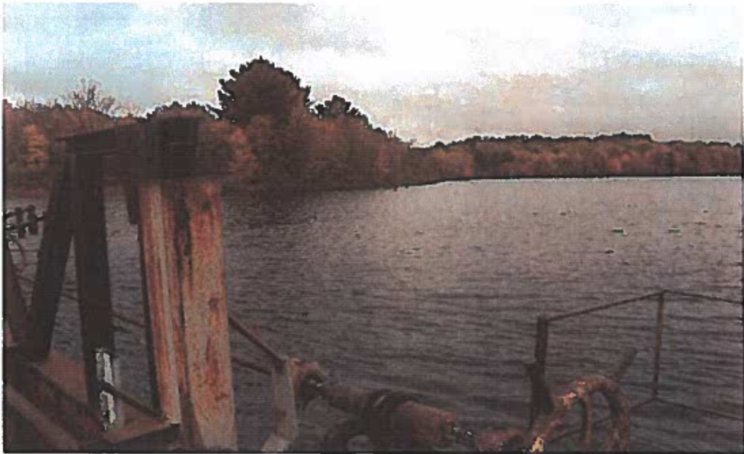
View from dam.
